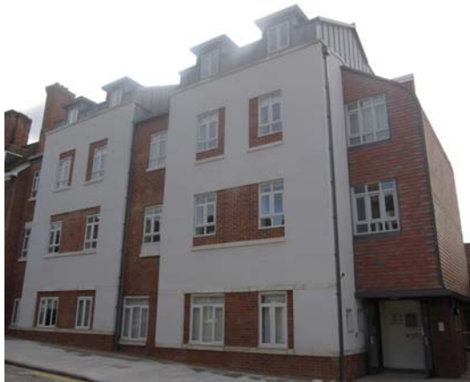
PHOTO 5 below: October 2011 - Alabaré Place is completed
