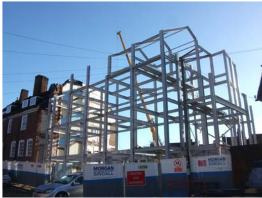
PHOTO 3 below: February 2011 - the steel frame is erected
